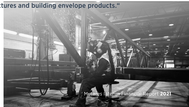
Manufacturing parts for a highway bridge
