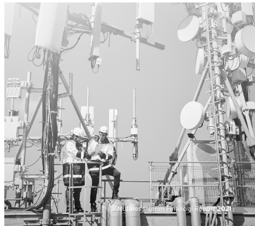
Employees during maintenance on site
